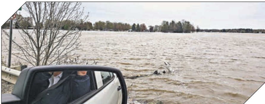
Midland Fire Department Chief Chris Coughlin and Assistant Chief Josh Mosher drove up to Wixom and Sanford lakes on Tuesday, May 19, 2020 to assess conditions. They saw how the water levels were nearly overtopping the earthen works at both dams. Despite the dam spillways flowing at capacity, the water continued to rise. (Photo provided/Chris Coughlin)
