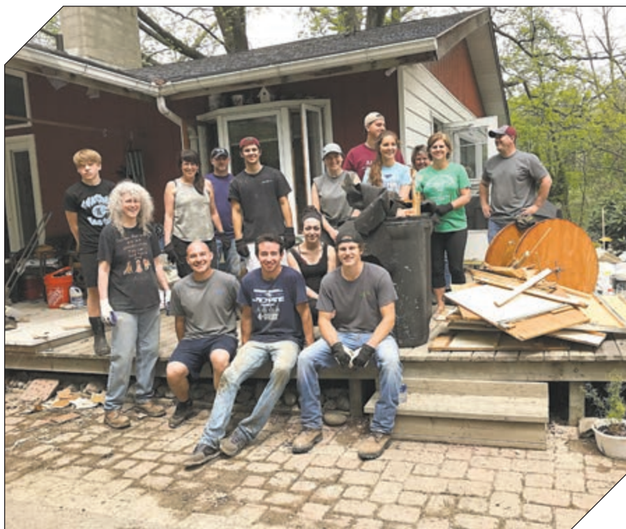
Linda and Wayne Allen, of Sanford, reported that so many people the couple didn't know just began showing up to help them muck out mud and debris, strip down drywall, pull up flooring, and haul things away.
