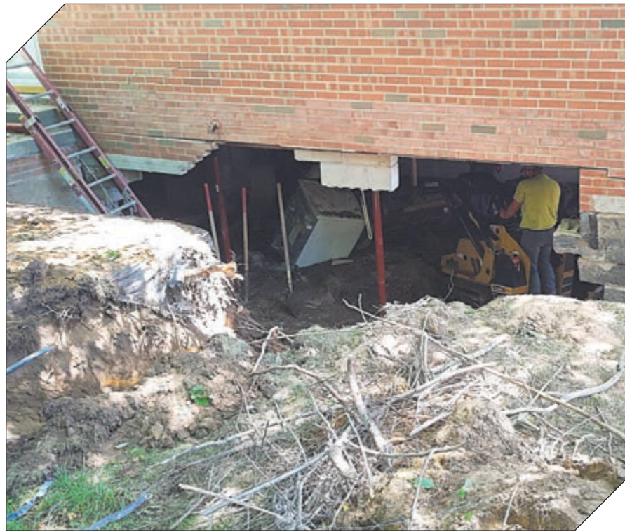
After the flood waters from the dam failures receded, Phillip Blaisdell, of Midland, was able to return to home. “When we walked up, we noticed that our basement windows had been blown out and the basement was full of water,” Blaisdell said. “The walls of our basement had also been blown out and the home was only supported by the corners of the foundation. A very surreal site to see.”
