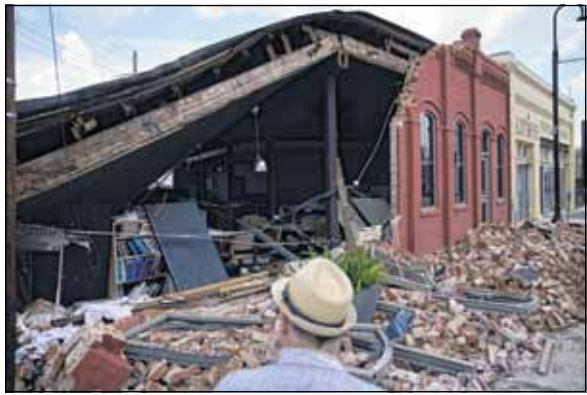
AP Photo/John Locher A man looks at a partially collapsed building Saturday in the aftermath of Hurricane Ida in Houma, La. Full restoration of electricity to some of the hardest-hit areas of Louisiana battered by Hurricane Ida could take until the end of the month, the head of Entergy Louisiana warned Saturday.
